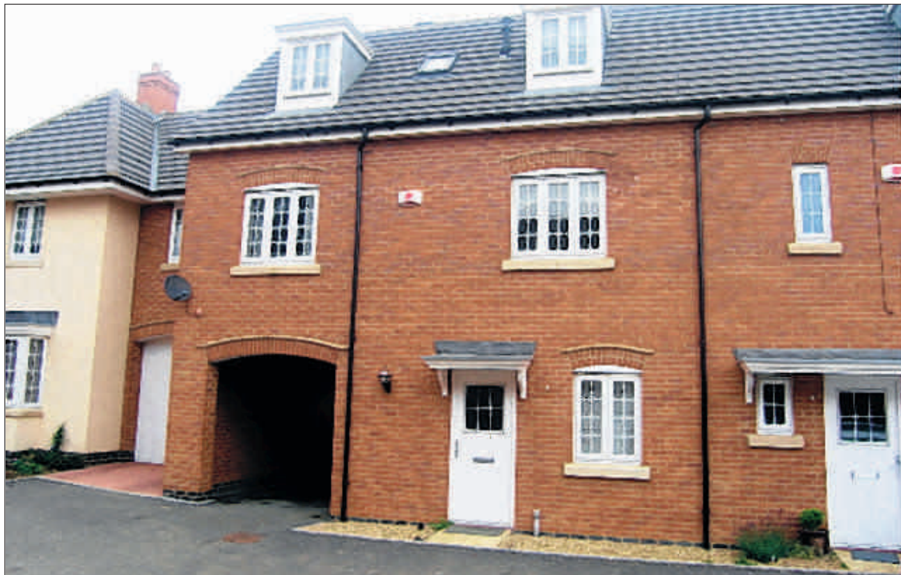
GAS CENTRAL HEATING: The three-storey property at Gateway Gardens.
